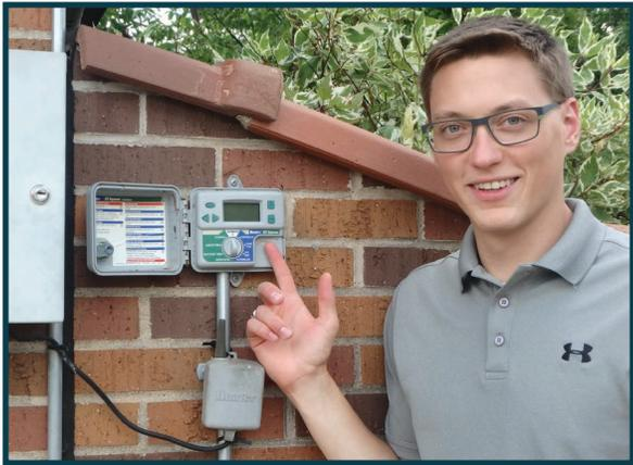
are set to water on certain days a week for an arbitrary amount of time. ET controllers utilize local weather data and landscape characteristics to determine if the property needs to be watered. The savings will vary based on weather, but a test site has seen a 49% reduction in water use since July 15th by switching from a clock-based to ET controller while maintaining and improving upon turf health and aesthetics.
